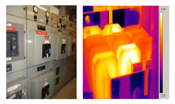
The thermal and ultrasonic scanning program has provided detailed information on the status of critical electrical equipment allowing our client to plan their maintenance and upgrade activities.
